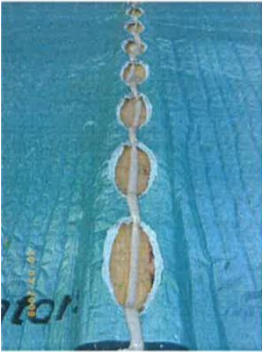
84% CONTINUOUS 5mm ADHESIVE BEAD FOR FLOORING (COMPLIANCE)
