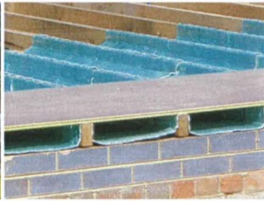
CONTROLLED LOCATION EVERY TIME ➤ GUARANTEED PUBLISHED R-VALUES ➤ CONTINUOUS VAPOR BARRIER ➤ INSTALL FLOORING AS NORMAL
