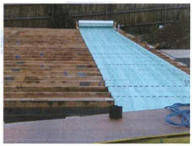
PATENTED OVAL SHAPED HOLES ACROSS THERMO FLOOR ALIGN WITH STANDARD JOIST SPACING
