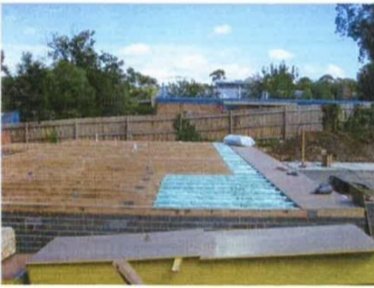
INSTALL IN-LINE WITH & SAME TIME AS FLOOR ➤ COMPLIANT, NON SQUEAKY FLOORING ➤ NO DAMAGE TO INSULATION ➤ NO PERFORMANCE LOSS ➤ SAFE WORKING PLATFORM + GROUND ACCESS
