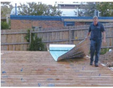
SIMPLE OVER-JOIST INSTALLATION AFTER SUB-FLOOR CONSTRUCTION & SERVICES INSTALLATION
